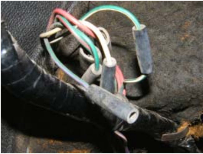
Figure 7. Here's a shot of the green purple stripe wire, just before it heads behind the kick panel.
