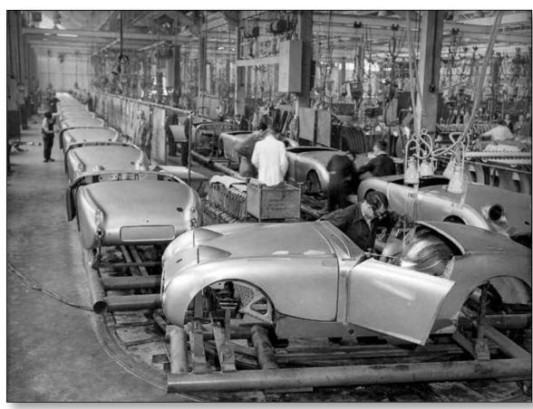
assembly line picture. At the end of the process, a complete body-in-white had been produced and was ready for transport to the Morris plant in Cowley.
